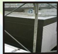
Wall Before Tiling
