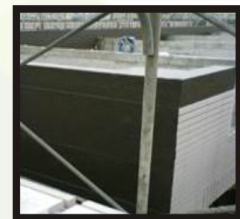
Wall Before Tiling
